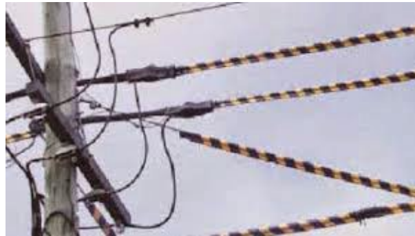
De-energise / installation of tiger tails
